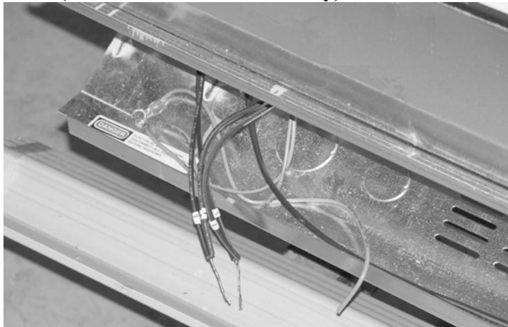
1. Refrigeration fan motors are labeled with the numbers 3 and 4.
