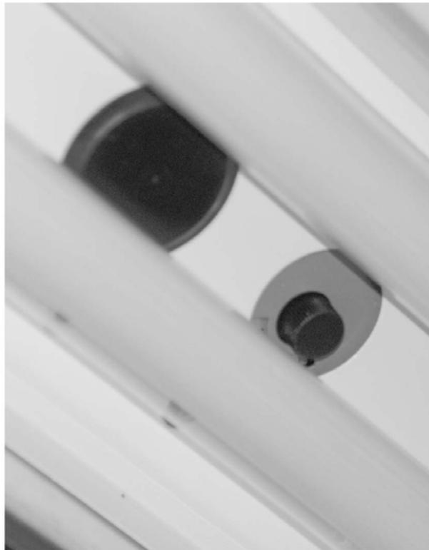
1. Ensure the fluorescent lamps located in front of the thermostat control have been removed.
