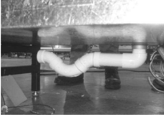
The drain pipe is installed on the outside-bottom of the case.
