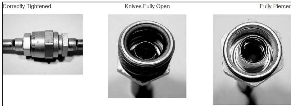
**NOTE:** Couplings that are screwed together but have threads showing are not only leaking refrigerant, but they are also restricting the flow of refrigerant through the small slits in the membranes or diaphragms.
