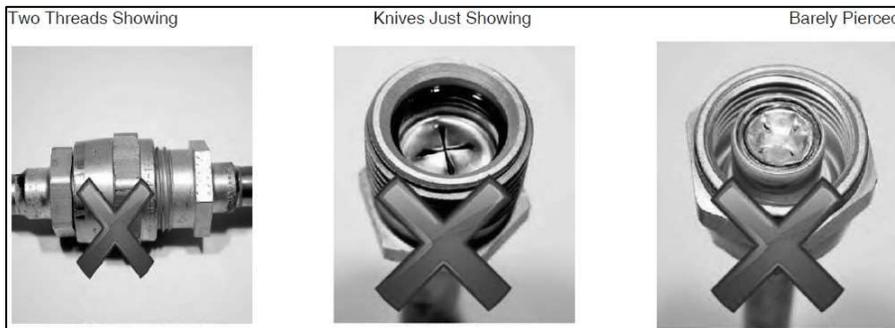
Below shows an even more complete assembly, with only one thread showing. However, this assembly is still not complete. If not tightened further, there will be refrigeration restrictions and leaks.
