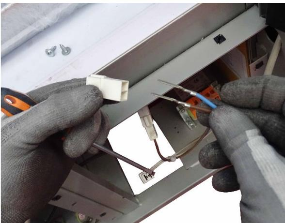
6) Unscrew and remove the electric components panel.
